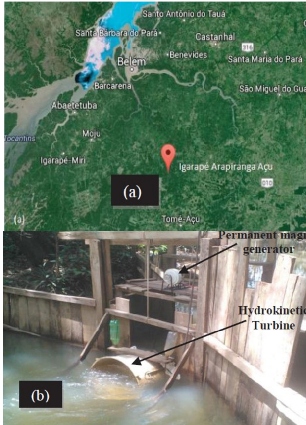
Figure 4: (a) Location of the small turbine in state of Pará, Brazil. (b) Details of the turbine installed at Arapiranga-Açu river.
